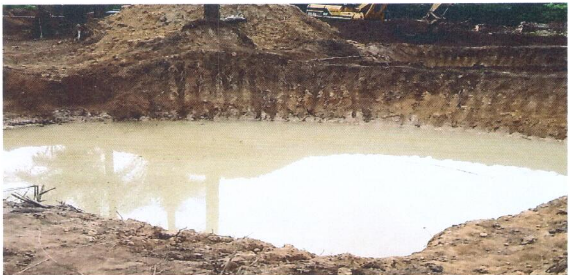
Plate 5: Picture of Excavated pits after manual recovery of oil
