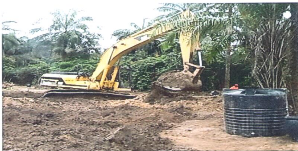
Plate 6: In –situ Homogenization process
