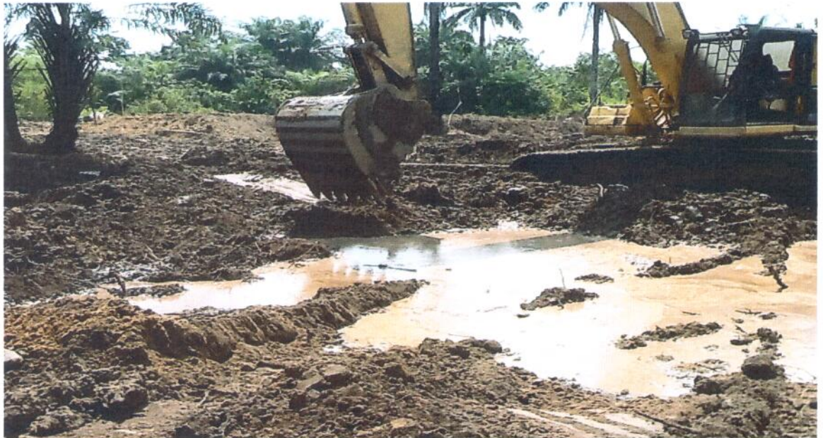
Plate 9: Excavator Backfilling pits after recovery of free oil.
